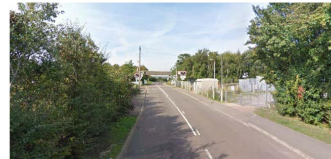
A421 at Stewartby at Green Lane access
