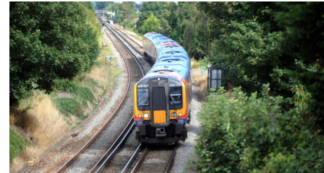
Marston Vale Train Line
