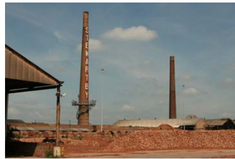
Stewartby Brick Works
